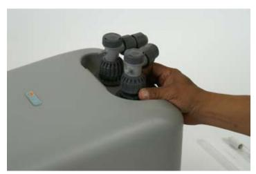
Unscrew the Ring Nuts and remove the shut off valves from the chiller.
